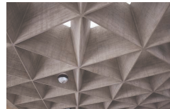
A roof in an airport where the structure is made stronger by using triangle shapes.
