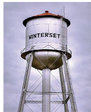
A support structure holding up a water tower. 8
