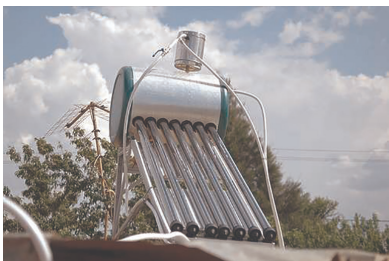
A solar water heater on the roof of a house. The water is in the tank. 5
