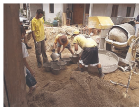
Mixing concrete using a mixer.
