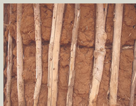
The wall of a mud house with a stick frame. 1
