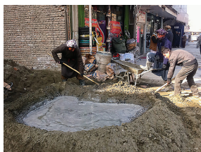
Mixing concrete using spades.
