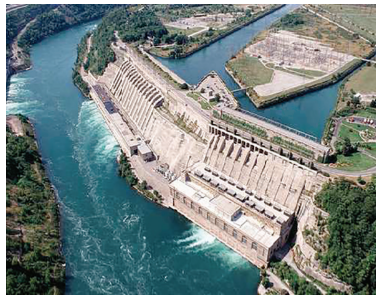
A large hydroelectric power station. As the water flows from the higher dam, through the station to the lower dam, electricity is made. 5
