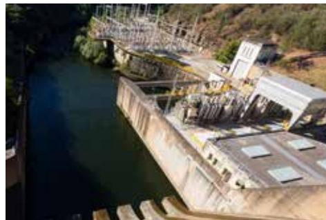
Figure 18.10: The water flows out the bottom of the power station and continues down the river.
