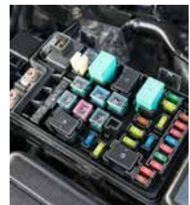
Figure 17.5: Motor cars also have fuses. Can you see the fuse in this photo showing the battery in a motor car?
