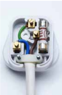
Figure 17.11: The three wires that form the cable leading to a plug.
