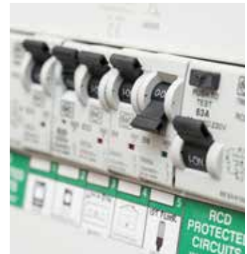
Figure 17.8: An example of circuit breakers showing the switches.
