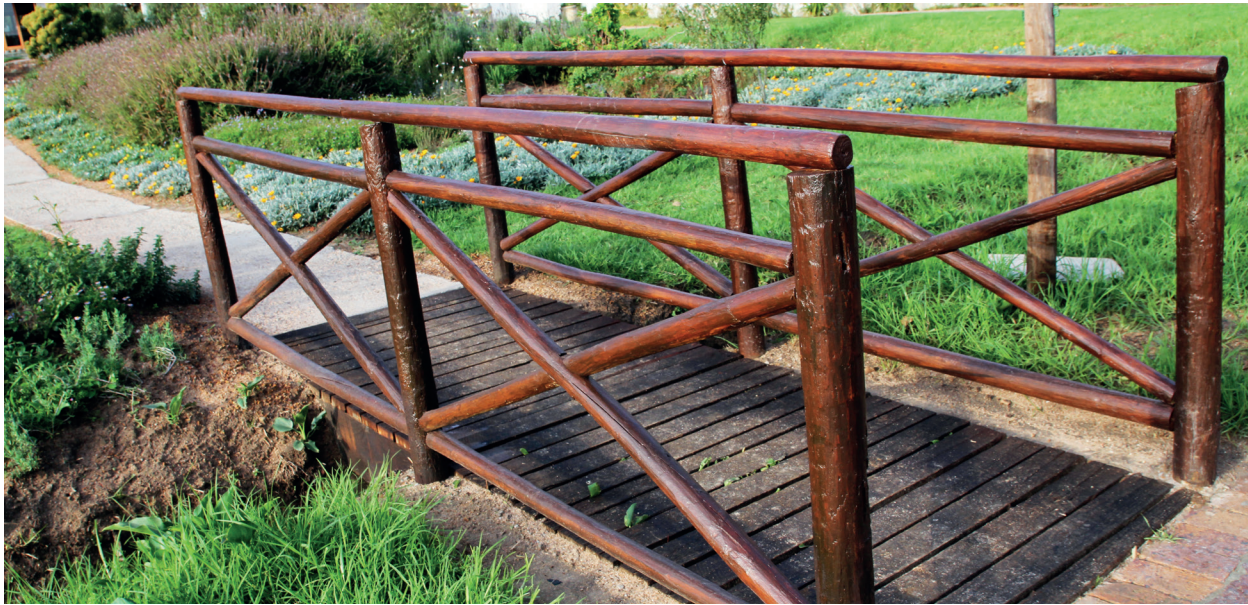
Figure 5: The bridge spans the stream.
