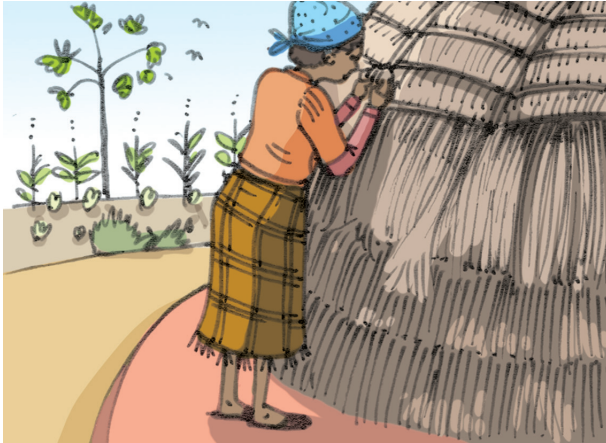
Figure 5: The framework is covered with grass.
