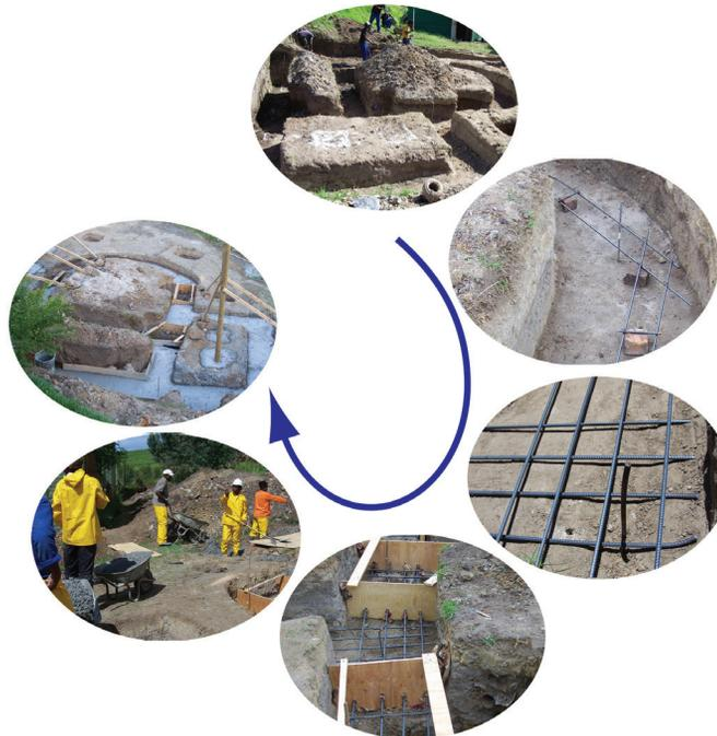
Figure 18: Steel reinforcement is used to strengthen the concrete foundations of a new house.
