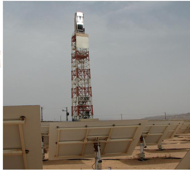
Figure 10: Thousands of mirrors at a solar thermal power station all reflect sunlight onto a tank on top of a tower. That is why the tank is shining so brightly.
