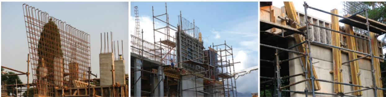
Figure 20: Steel reinforcement is placed inside a concrete wall of a big building.
