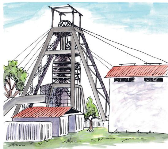
Figure 4: The headgear of an underground mine. The shaft goes straight down into the ground under the wheels of the headgear, sometimes kilometres deep.
