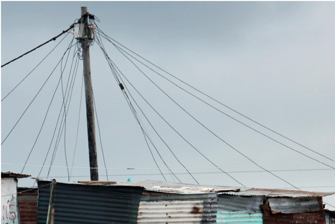
Figure 5: An informal community with an electrical supply. Notice the control boxes at the top of the poles. They control how much electricity each household uses and have a built-in safety mechanism for when there is a short circuit.
