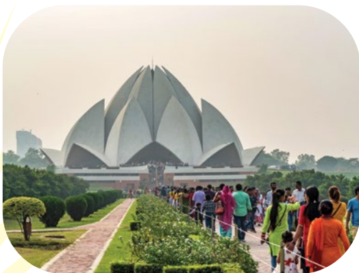
g. The Mashriqu'l-Adhkár in Delhi, India. It is a Bahá'í House of Worship , or temple. It has nine entrances so people can enter from any direction.
