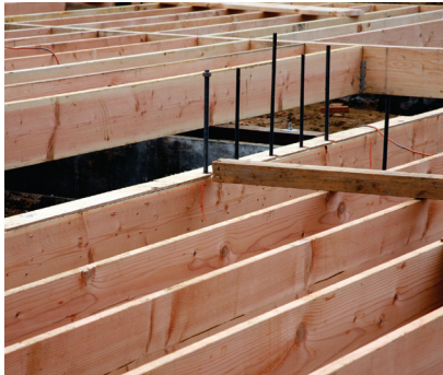
Figure 3.24a Wooden floor joists
