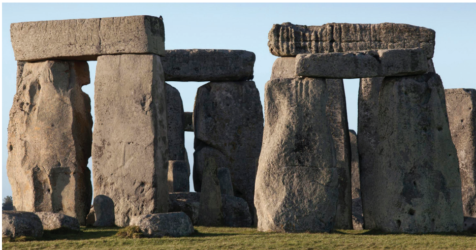
Figure 5.8 Ancient beams were usually simply supported.
