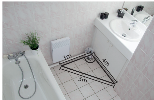
Figure 1.9 Using the 3-4-5 technique
