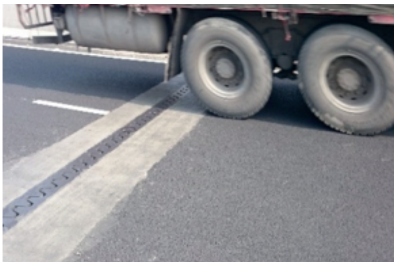
Figure 5.9 Expansion joints on a bridge
